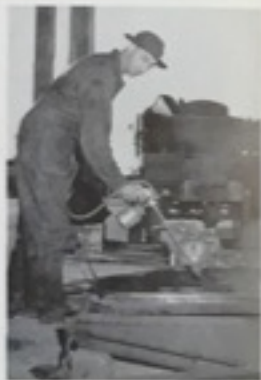
Equipment is painted
