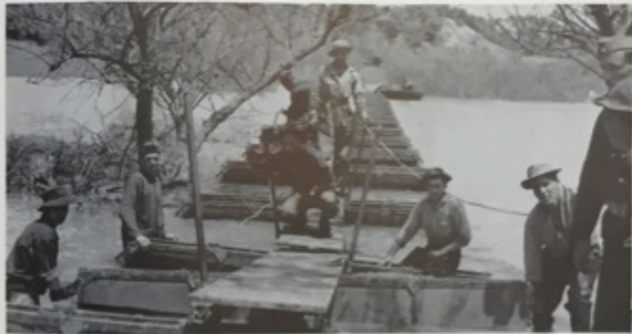
Pontoons used in floating trestle bridge.
