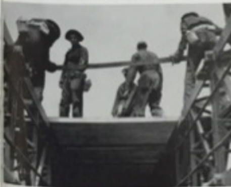
Docking the portable steel bridge.
