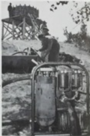
Constructing portable water purification plant.
