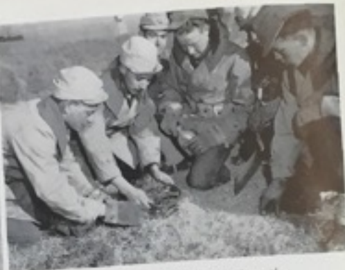
One of the early stages of destruction. Planting a steel mine.
