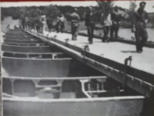
The finished product of hard work—a light pontoon bridge.
