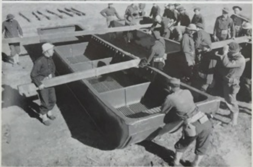
Ponton Bridge in the Making
