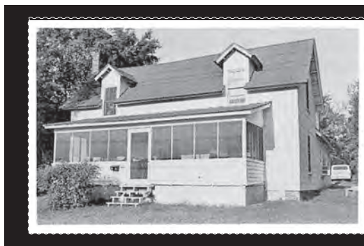
The house at 507 North Greensboro was lost to a fire in 2000.
