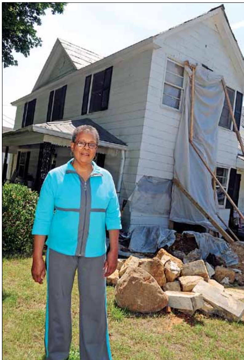
Delores Clark in front of her home, where her chimney fell when workers attempted to repair it. Clark's grandfather, a freed slave, built the house.
