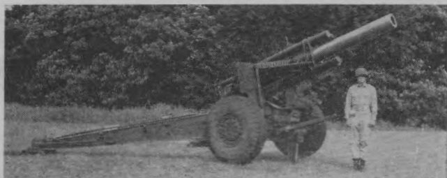
Figure 90. The 155-mm. howitzer M1, carriage M1A2. Weight—12,700 pounds. Weight of projectile—95 pounds. Range—16,355 yards. Rate of fire—2 rounds per minute.
