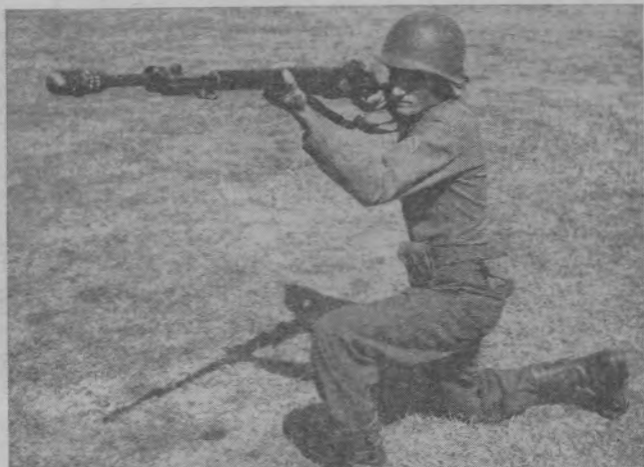
Figure 70. The rifle grenade. Weight—1¼ pounds. Range—365 yards. Effective killing radius—10 yards.
