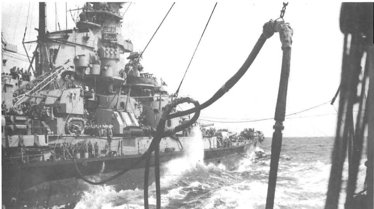
A SOUTH DAKOTA-class battleship fuels from an oiler. She, in turn, will extend the reach of her task group by replenishing screening destroyers.
