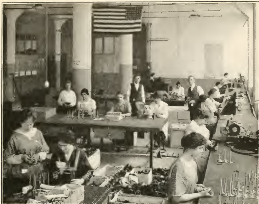
INSPECTION OF VALVES FOR LIBERTY ENGINES, PACKARD COMPANY.
