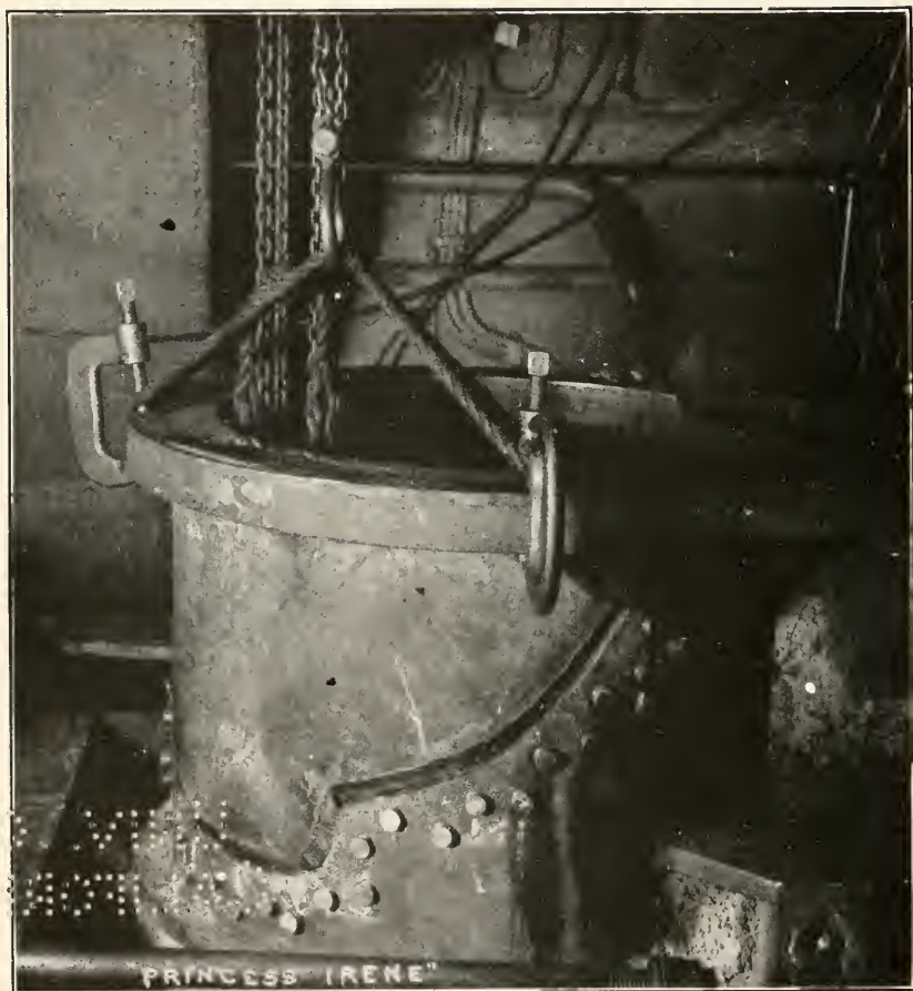
PRINCESS IRENE, H. P. CYLINDER; INSERT IN PLACE READY FOR WELDING.
