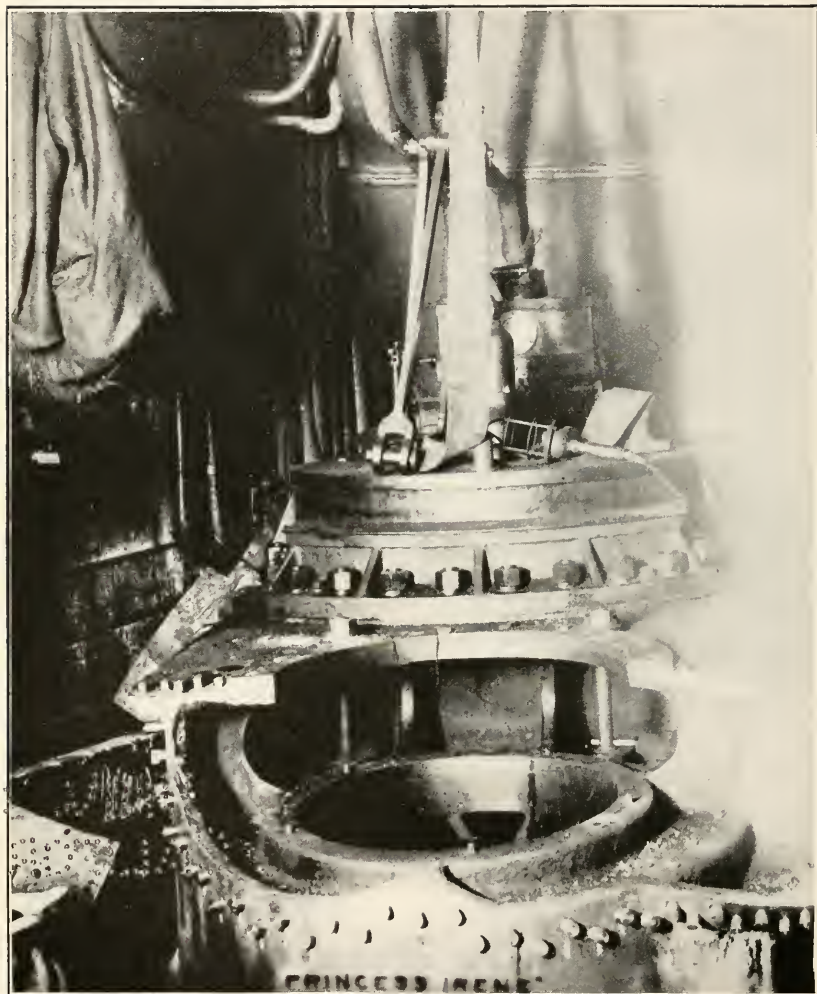
PRINCESS IRENE, BROKEN I. P. VALVE CHEST.
