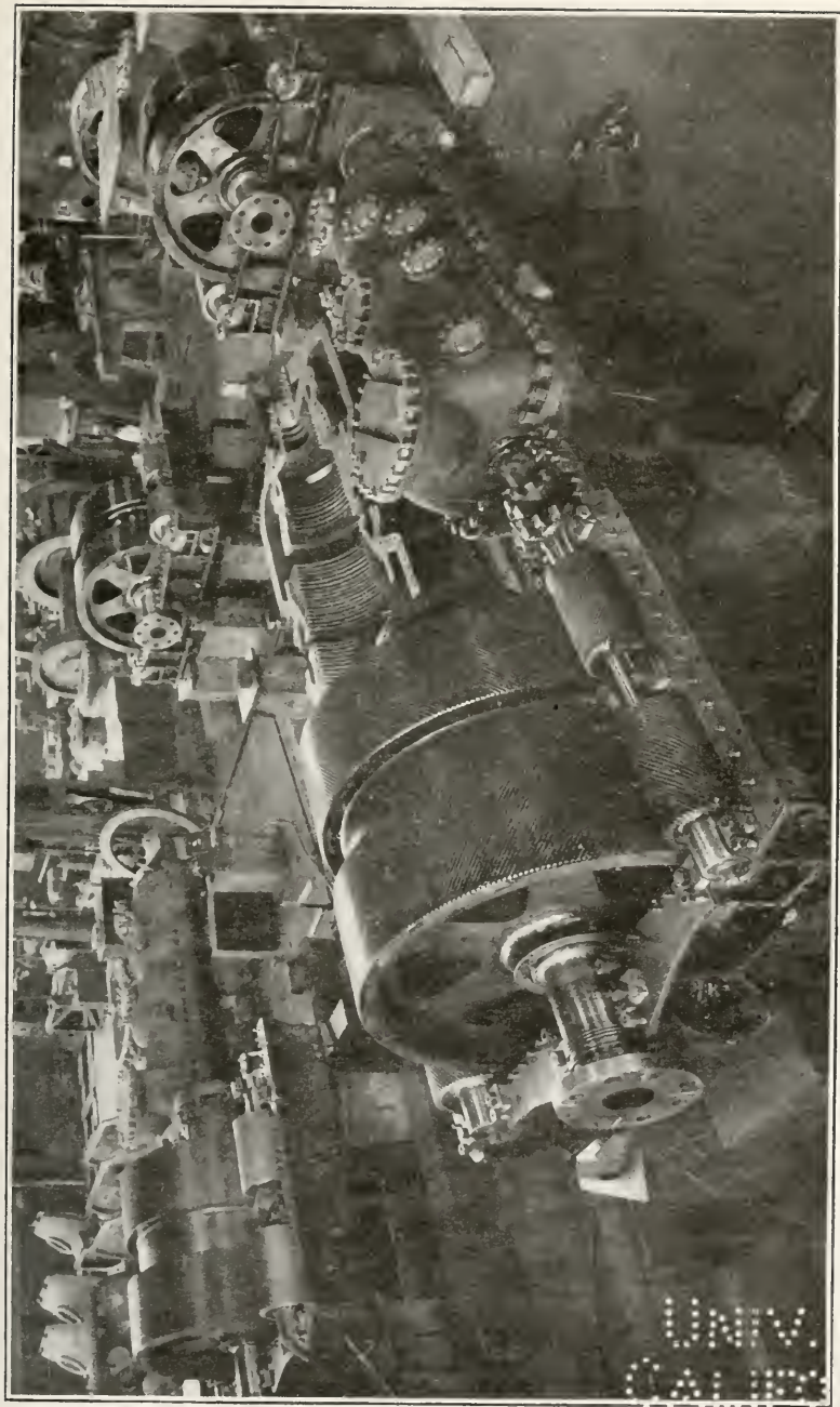
PARSONS TURBINES AND REDUCTION GEARS AT CRAMP'S.
