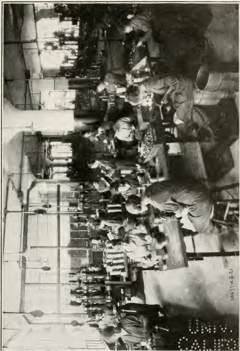
MANUFACTURING WORTHINGTON PUMPS FOR DESTROYERS.
