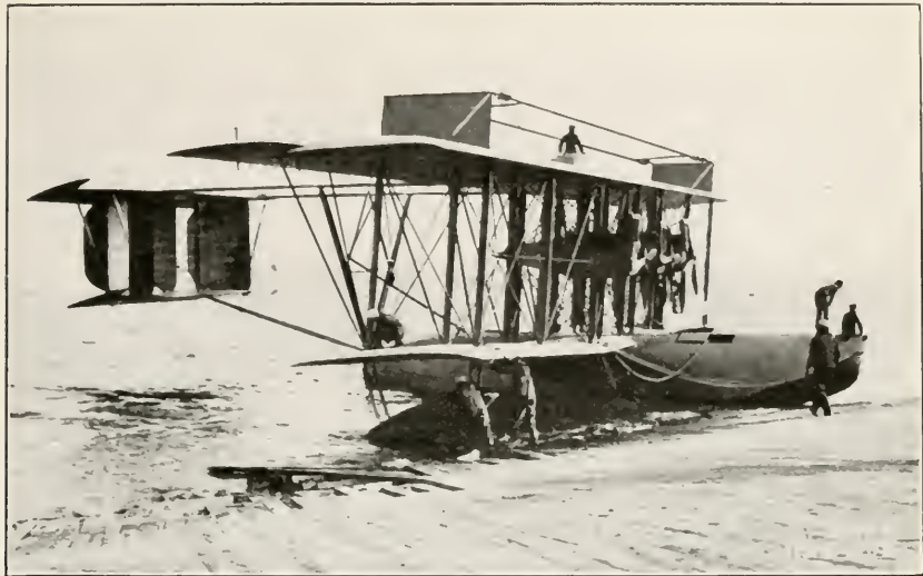
FIG. 21.—SEAPLANE, SHOWING SKID FIN ANTENNA.
