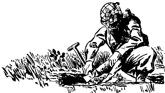
SPOIL BEING REMOVED CORRECTLY
