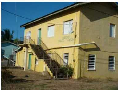
Hopkins Police Station showing significant structural damage to back staircase and support columns due to the use of sea sand in construction
