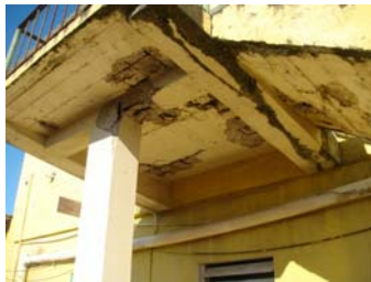
Hopkins Police Station showing significant structural damage to back staircase and support columns due to the use of sea sand in construction
