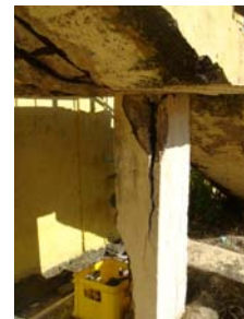
Hopkins Police Station showing significant structural damage to back staircase and support columns due to the use of sea sand in construction
