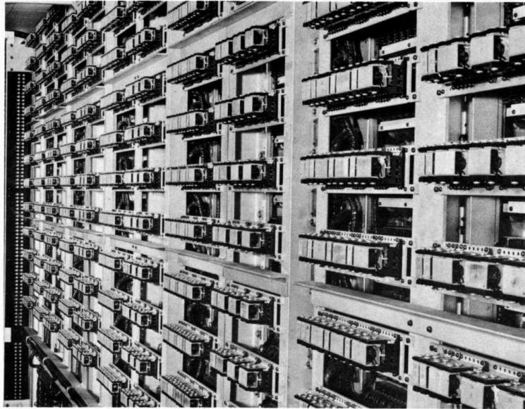
X Storage Counter Relays
