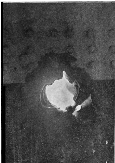
Shot-hole in Port Bow of the Texas , made by a Six-inch Shell (photographed from the inside).
