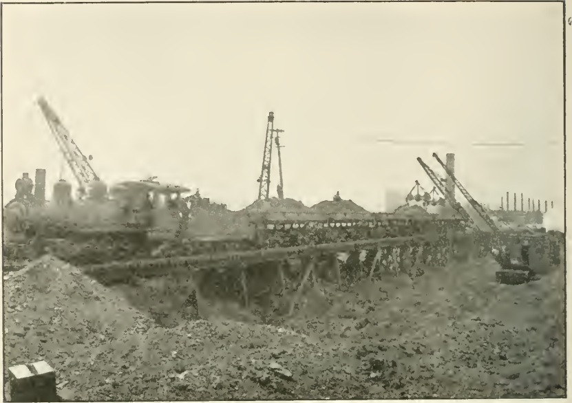
Loading train for delivery of coal to barges, Emergency Fuel Depot, Constable Hook, N. J.
