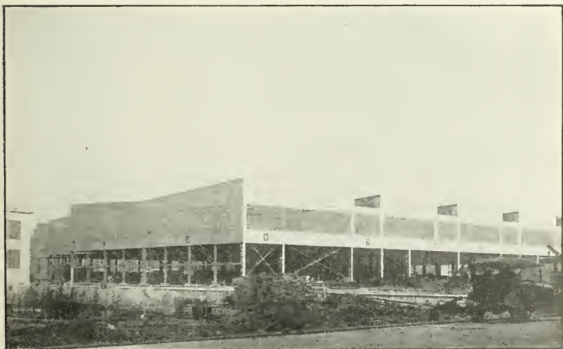
Steel-storage shed, Navy Yard, Norfolk, Va.
