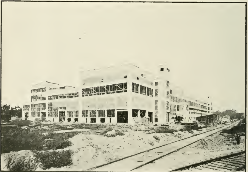
Structural shop, Navy Yard, Mare Island, Calif.
