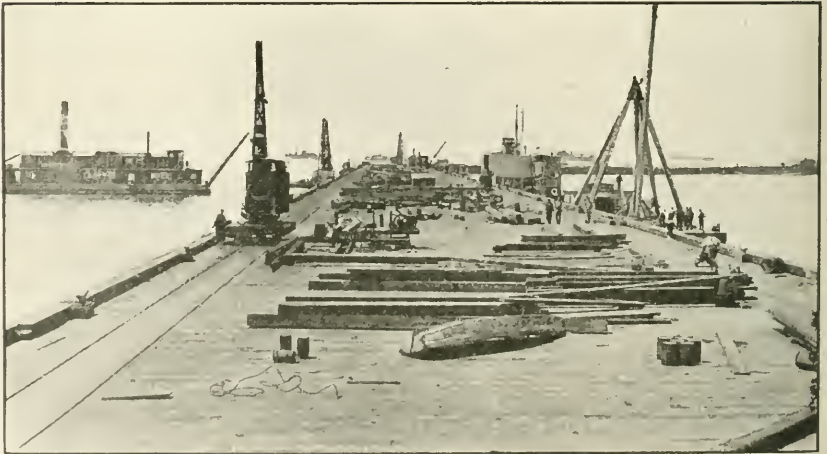
Construction of pier at south of submarine basin, Naval Operating Base, Hampton Roads, Va.
