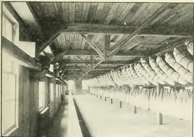
Interior view of quarters, Wissahickon Barracks, Cape May, N. J.
