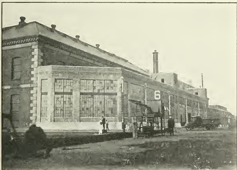
Foundry, Navy Yard, Boston, Mass. Second extension.
