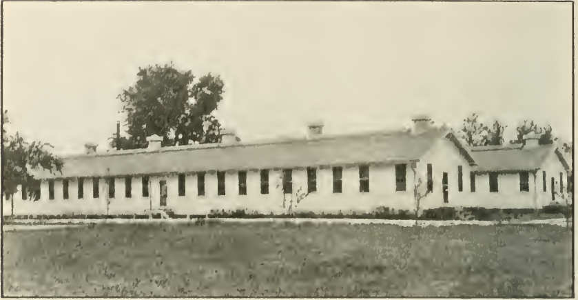
Ward buildings, Naval Hospital, New Orleans, La.
