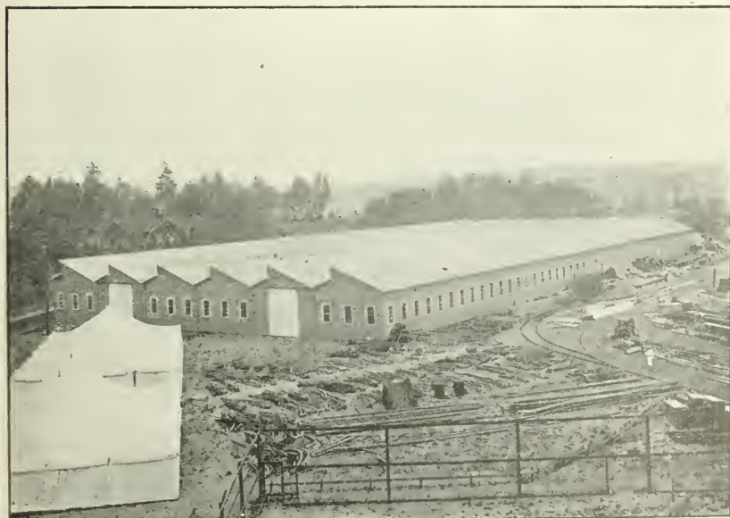
Temporary general storehouse, Navy Yard, Puget Sound, Wash.
