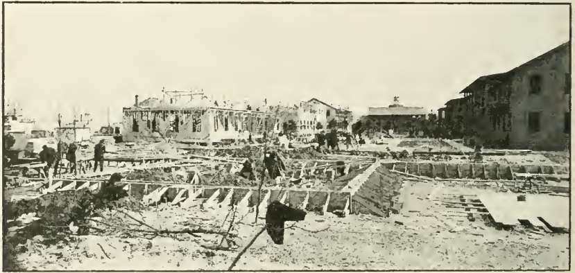
Barracks and mess-hall, Naval Air Station, Hampton Roads, Va.; view of court.
