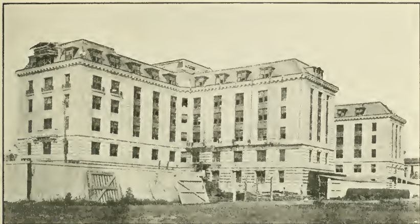
Bancroft Hall extension, east wing, Naval Academy, Annapolis, Md.
