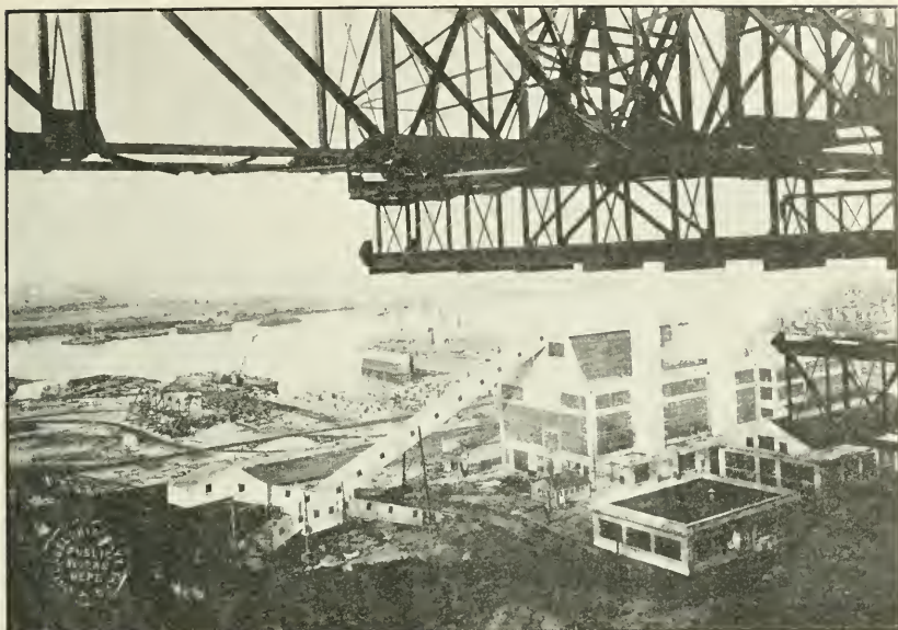
Power plant, Navy Yard, Philadelphia, Pa. View showing coal-handling plant (left), taken from crane runway of shipbuilding slip.
