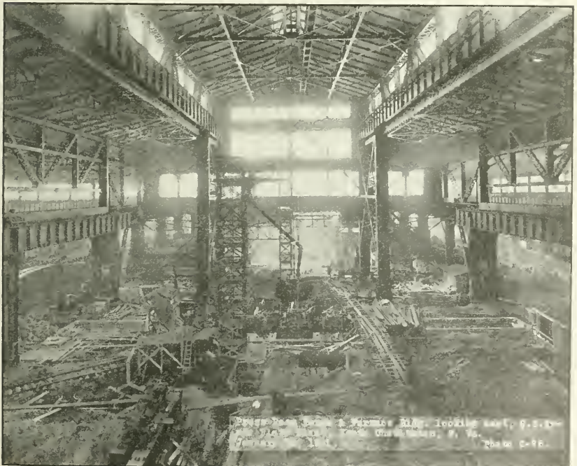
Press room, forge and furnace building, Armor Plant, Charleston, W. Va.
