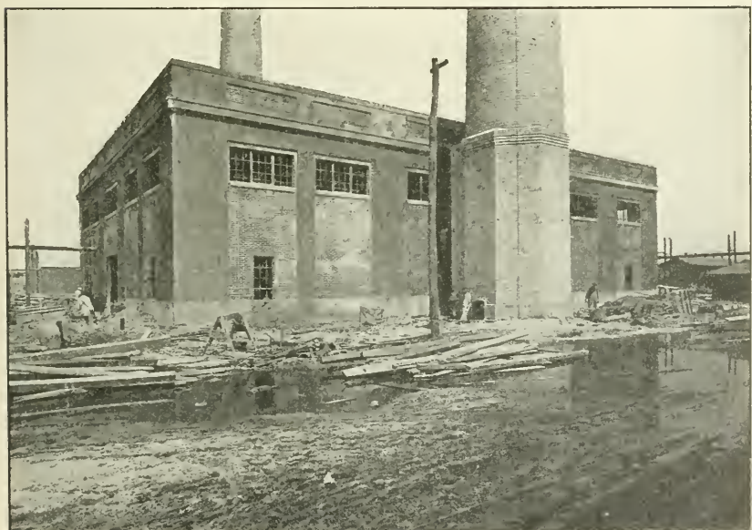
Boiler plant, East Camp, Hampton Roads, Va.
