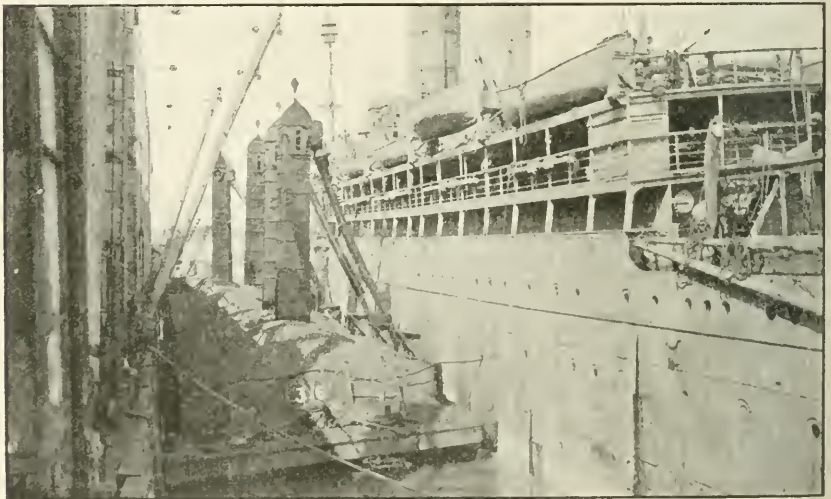
De Mayo elevators in operation at Bunkering Depot, Newport News, Va.
