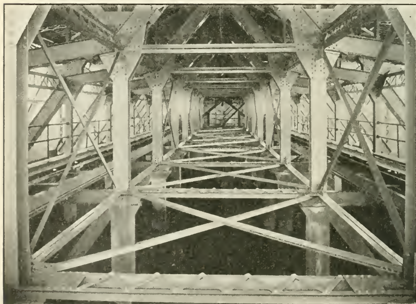
Overhead coal bunkers in power plant, Navy Yard, Philadelphia, Pa.
