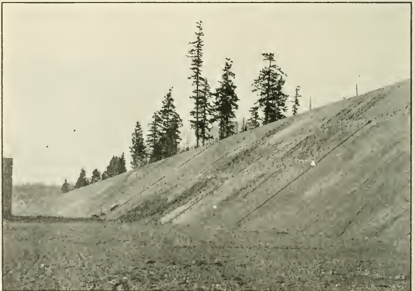
Grading operation completed, Navy Yard, Puget Sound, Wash. Slope protection.
