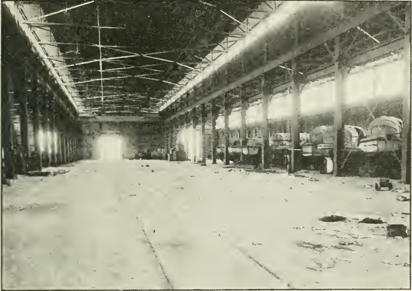
Partial interior view, boat and general storage building, Navy Yard, Philadelphia, Pa.
