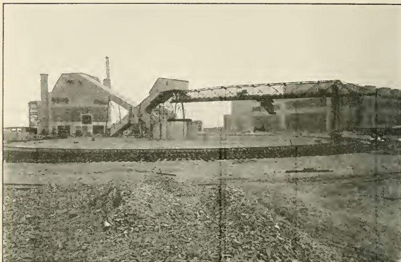
Coal-handling installation at power plant, Navy Yard, Philadelphia, Pa.
