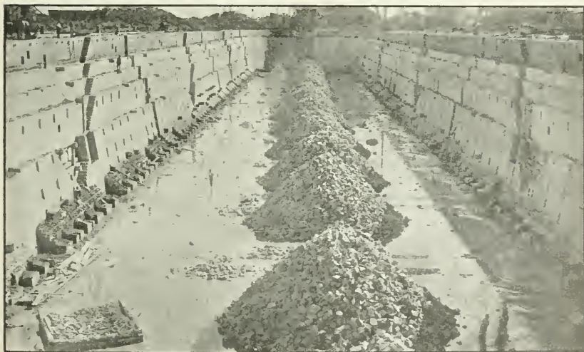
Dry Dock No. 1, Naval Station, Pearl Harbor, Hawaii. Interior view after first pumping, showing rock ballast before completion of floor.
