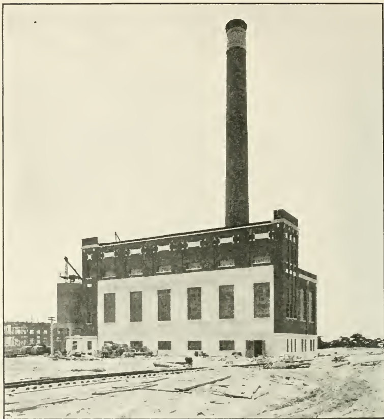
Boiler plant for industrial section of Naval Operating Base, Hampton Roads, Va.
