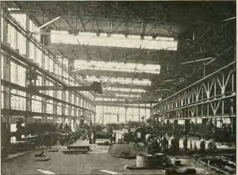
Structural shop, Navy Yard, New York, N. Y. Partial interior view.
