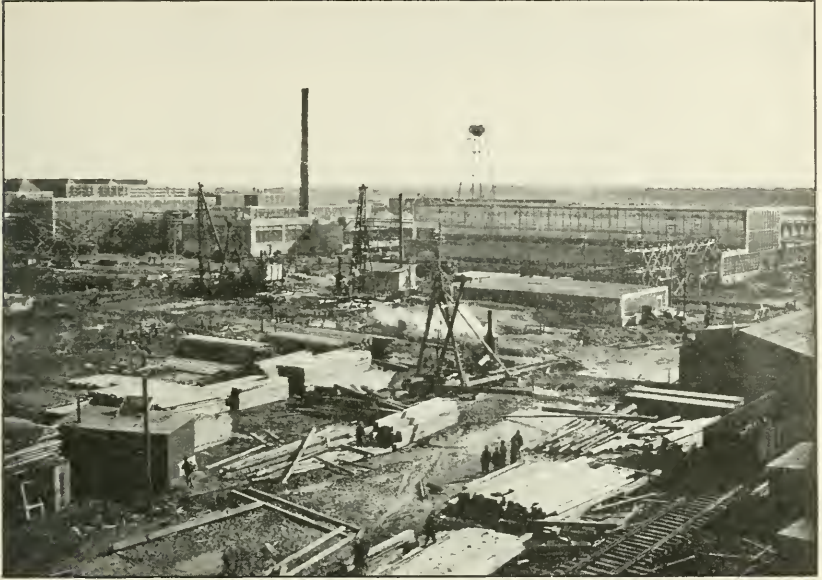
Squantum destroyer plant. General view during construction.
