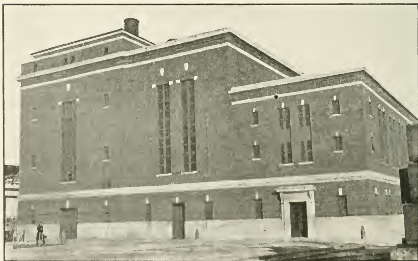
Power plant at Naval Torpedo Station, Newport, R. I.
