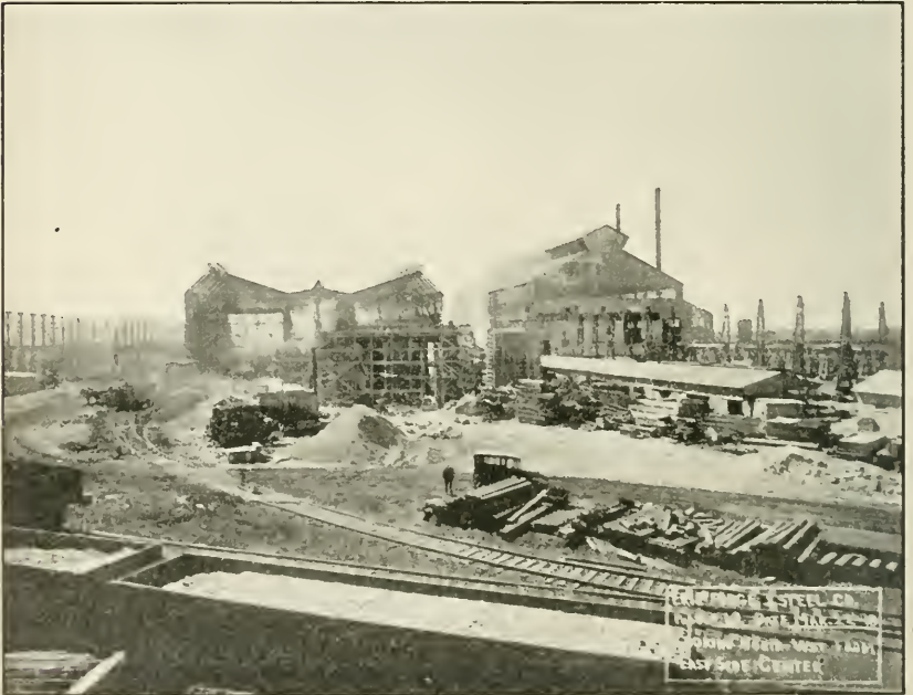
General view of Navy extension to plant of Erie Forge Co., Erie, Pa.
