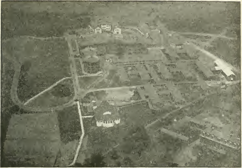
Seaplane view of Naval Hospital, Chelsea, Mass., showing emergency units.
