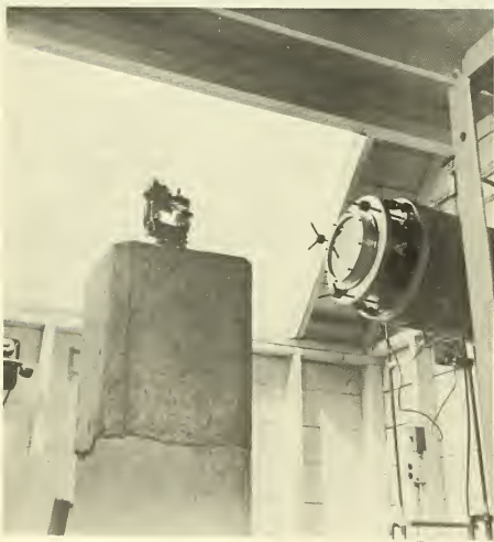
Figure 6 West Pier - Theodolite Mounted
