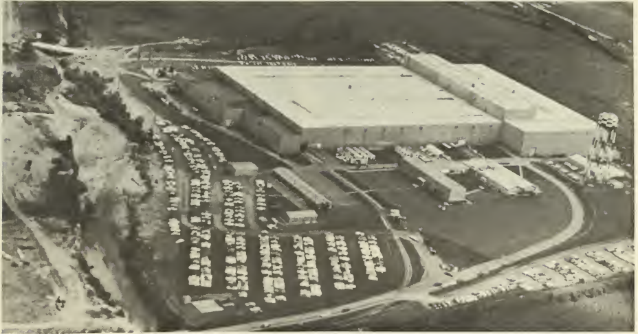
Figure 1 Aerial View of Facility
