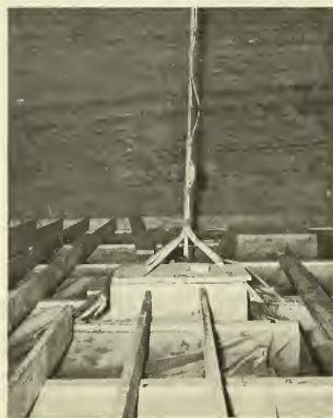
Fig.17 View of Joists & Foundation
