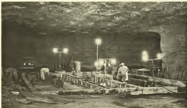
Figure 16. View of Footings
