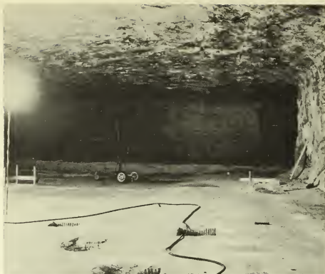
Figure 13. Holes in Salt and Bedrock for Pedestals
