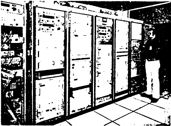
FIGURE 4.- ESTL TDRSS GROUND STATION EQUIPMENT.
