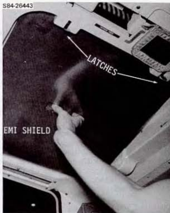
W8 EMI SHIELD INSTALLATION/REMOVAL
