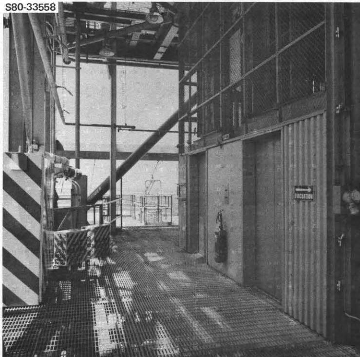
ELEVATORS - 195 FT. LEVEL
