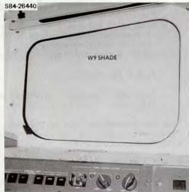
W9 SHADE (INSTALLED)
