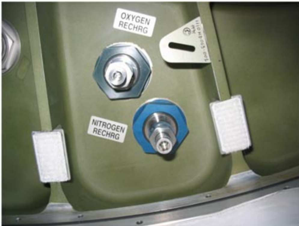
Figure 4. MLI and PTCS Interfaces on NOD2 Bulkhead (MLI removed).
