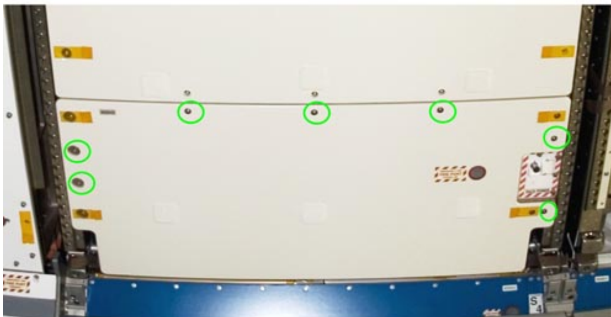
Figure 1. Example of lower closeout on Avionics Racks (Launch Restraint Bolts circled in green).
