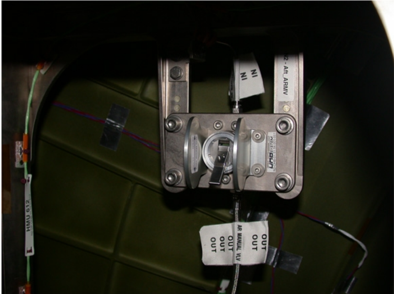
Figure 4. Node 2 Aft SDS Manual Valve.
