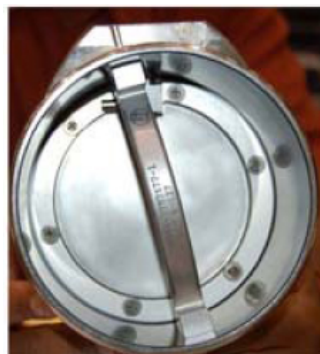
Figure 8. Example of Closed IMV Valve.
