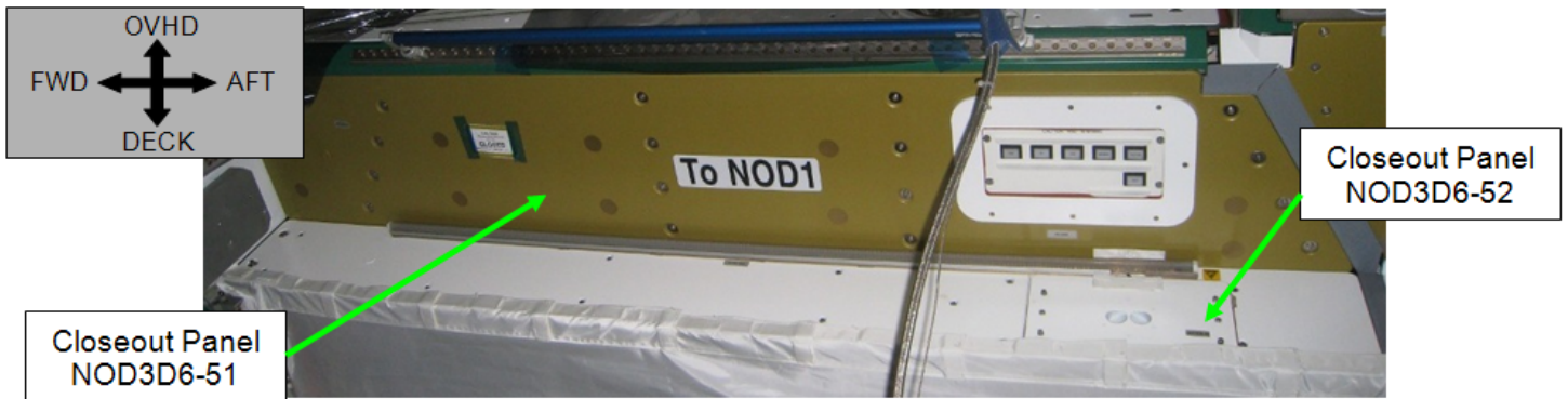
Figure 16.- Node 3 Starboard Endcone Deck Closeout Panels (looking Starboard).
