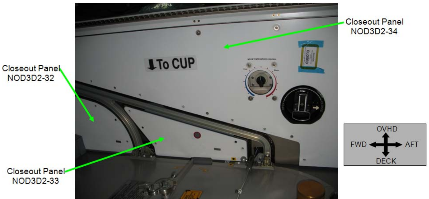
Figure 5.- Node 3 Deck Midbay Closeout Panels (looking Starboard).
