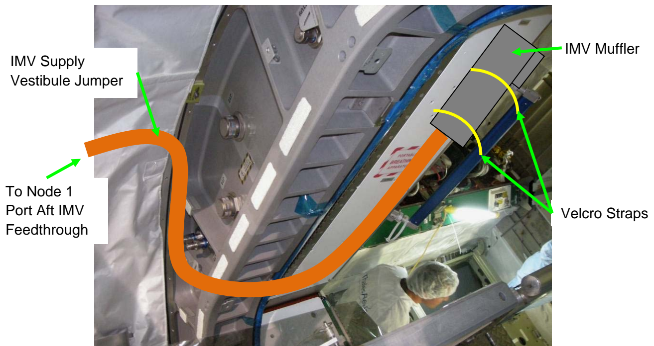
Figure 15.- IMV Supply Vestibule Jumper Temporary Install (View Looking Aft-Port).
