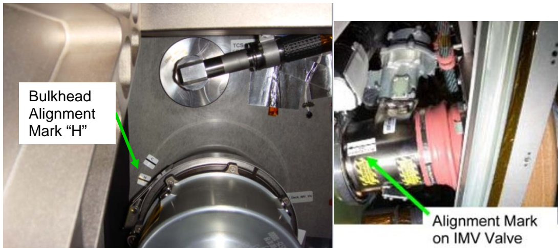
Figure 9.- Bulkhead Alignment Mark and IMV Valve With Alignment Mark.
