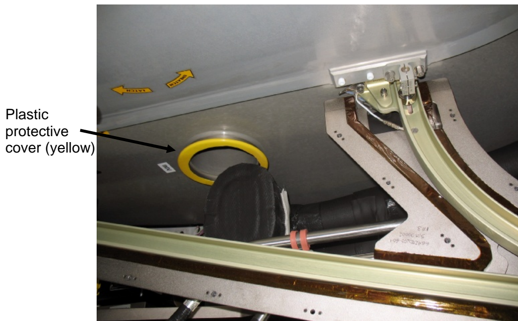
Figure 3.- Plastic Protective Cover Installed on IMV Feedthrough Flange.
