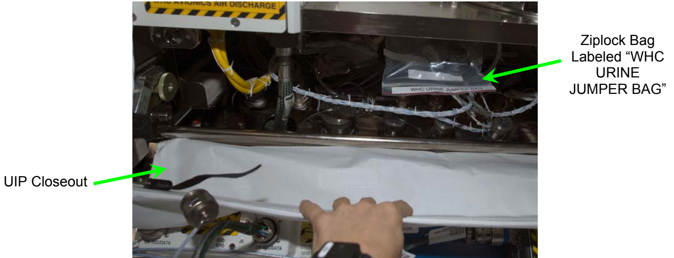
Figure 3.- WHC Rack UIP Closeout.
