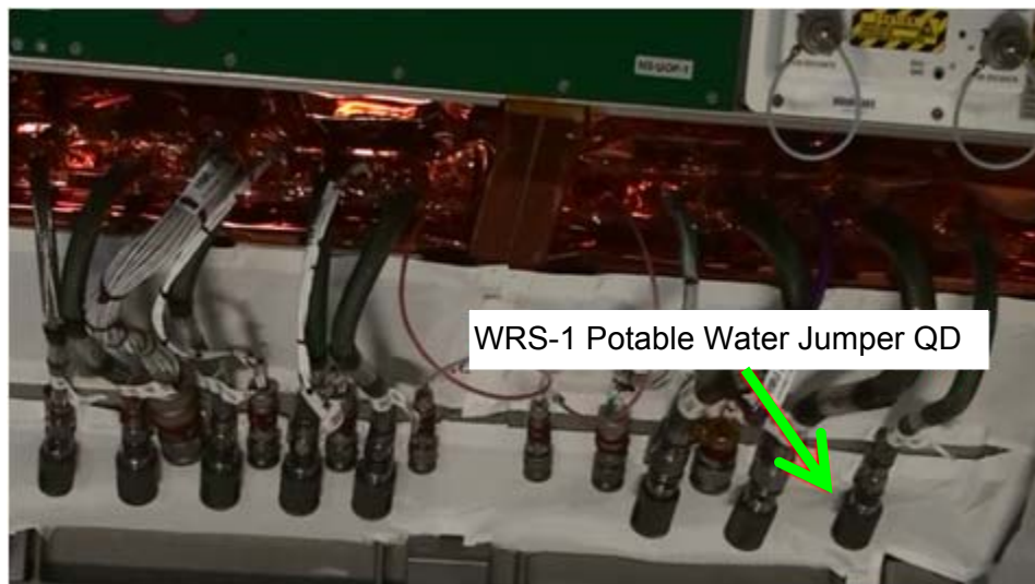
Figure 8.- NOD3D5 WRS-1 Umbilicals With WRS-1 Potable Water Jumper QD Pointed Out.
