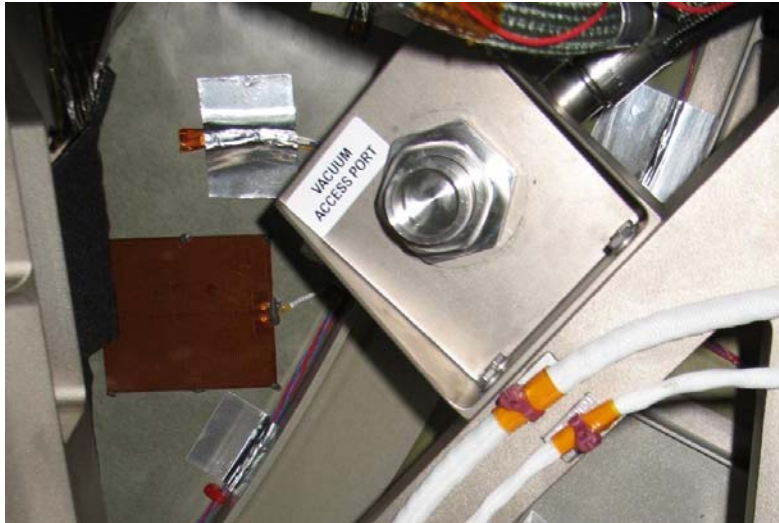
Figure 1.- Node 3 Vacuum Access Port
