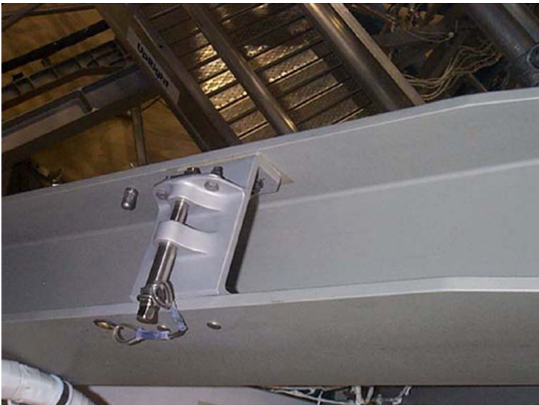
SARJ Brace Launch Restraint bolt (re-inserted into housing after brace release)
