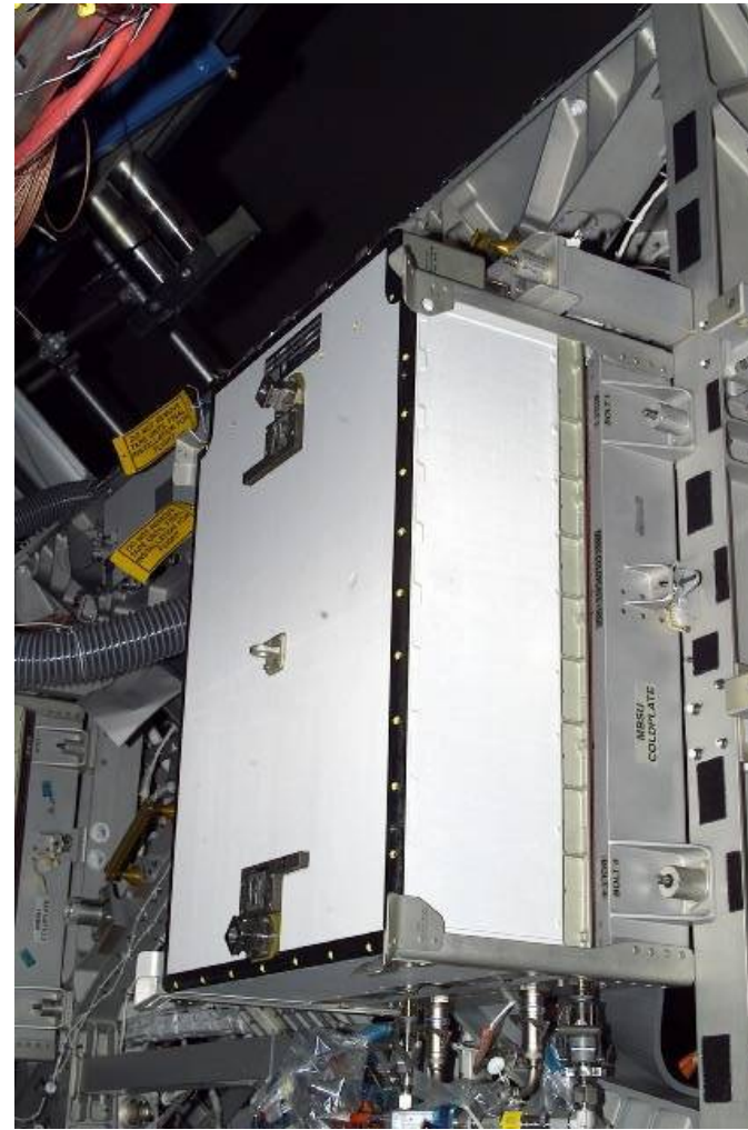
MBSU at worksite
