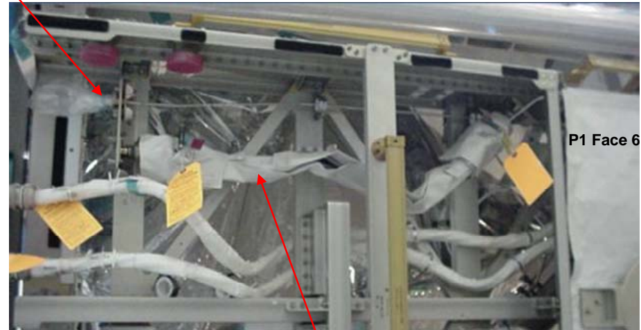
Fluid Jumper Install Location (M3)
