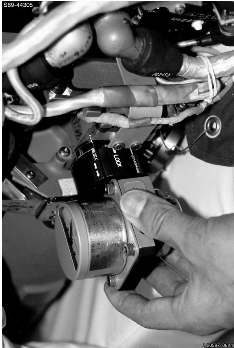
Figure 3.2-6. BTA installation on PPRV
