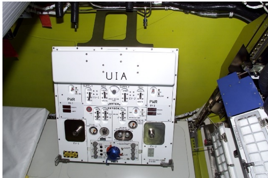
Figure 1.8-2. Back-up UIA installed
