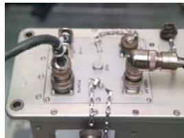
11 CAUTION: Ensure ergometer and power panel are OFF before making connections. Note: Steps will interrupt power to other loads on utility panel. Connect display panel to ergometer and connect Pre-routed power cable.
