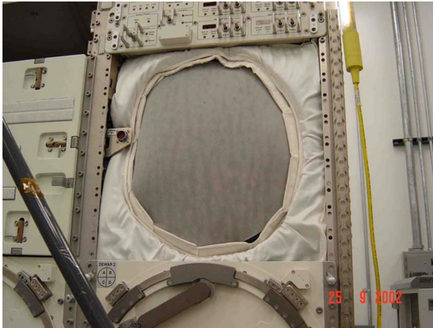
Figure 3.5-5: Acoustic protections in front of Brayton machine
