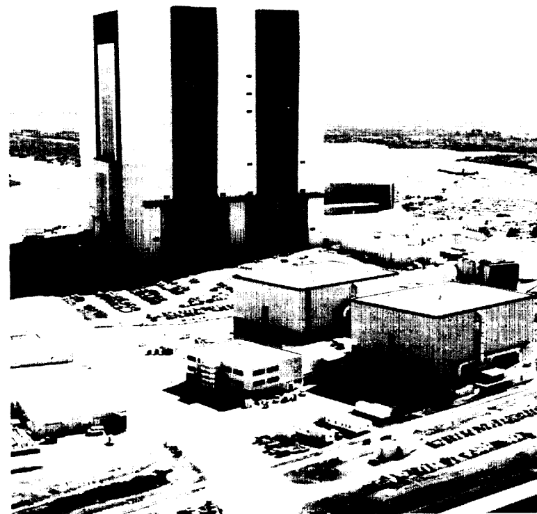
Orbiter Processing Facility with VAB in background
