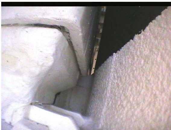
Borescope Dry-run at Pad A
