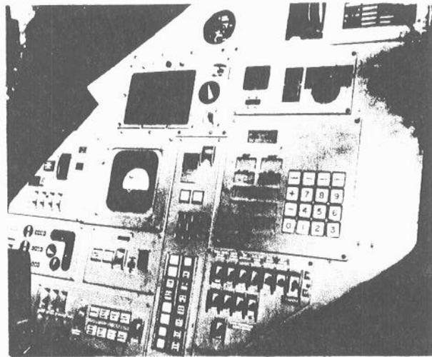
Fig. C12 G&N DSKY in NADC Gondola
