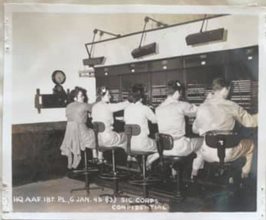
TELEPHONE SWITCHBOARD -- being operated by 424th personnel, from l. to r., Cpl Hampton, Cpl Schlundt, T/S Feiter, Cpl Flanner and Sgt. Savely.
