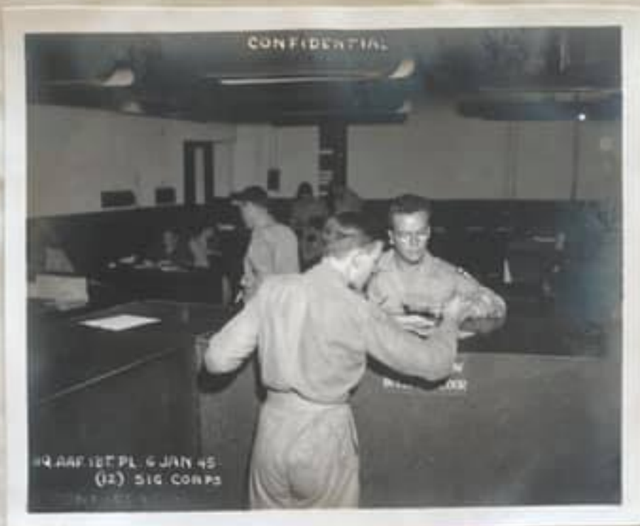
MESSAGE CENTER COUNTER -- Situated just inside the Signal Center, in the counter where members of British and other American Units at Hastings Air Base deliver and receive messages to and from New Delhi and other headquarters in the Theater, as well as to and from China and the United States. Pfc Dougherty gives service to a member of the British forces.
