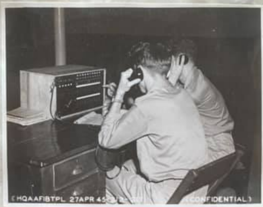
T/S Gwely, left, and Cpl Flanner operate the chief operator's booking board for long distance calls. Designed by W/Mgt Frank H. Wilcox, Wire Chief, this board enables the chief operator to keep a log on all long distance calls made.
