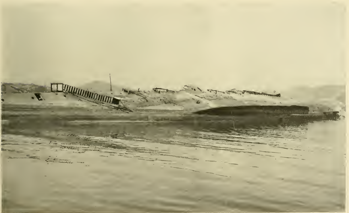
Photo 18 Hull View of Oyodo (CL)
