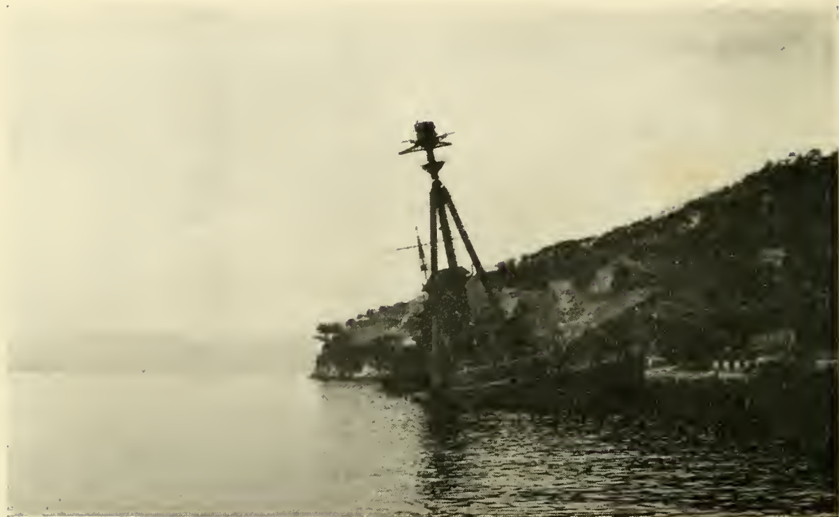
Photo 23 Port Quarter View of Superstructure of Settsu (CL)
