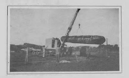
Method of pre-inflating pontoons and loading on dump trucks used in Roer Crossing.
