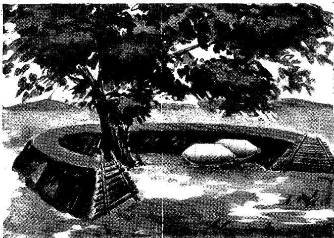
FIGURE 17.—Bomb storage in revetment.
