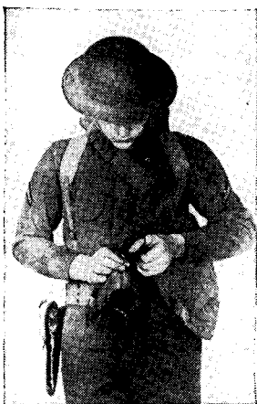
FIGURE 37.—INSPECT MASK. TWO. Examining outlet valve.
