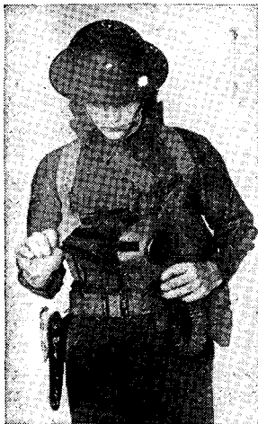
FIGURE 39.—INSPECT MASK. TWO. Examining head harness.
