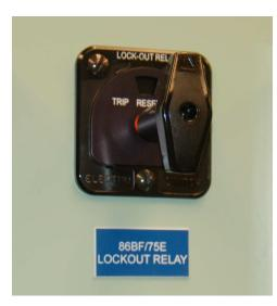
This lockout relay is shown in the "Reset" position, having been placed in that state by someone rotating the handle clockwise until it points vertically. When a remote signal energizes this lockout relay's trip coil, it moves by spring action into the "Trip" position, the handle turning about 45 degrees counter-clockwise and an orange "target" appearing just above the handle shaft. The lockout
