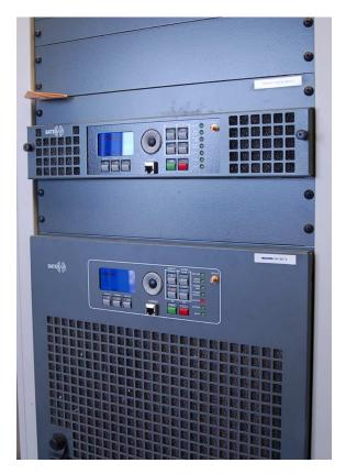
In this particular case the amplifier is rated for 20 kiloWatts of continuous RF power but typically operates at about 17 kW. The antenna array for this transmitter consists of three circular-polarized dipole antenna elements fed through a semi-rigid coaxial transmission line atop a tower approximately 100 meters in height.
