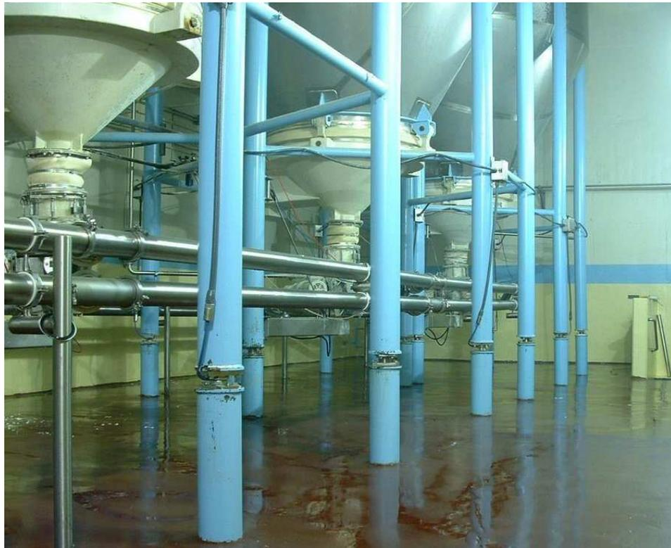
One very important caveat for weight-based level instruments is to isolate the vessel from any external mechanical stresses generated by pipes or machinery. The following illustration shows a typical installation for a weight-based measurement system, where all pipes attaching to the vessel do
