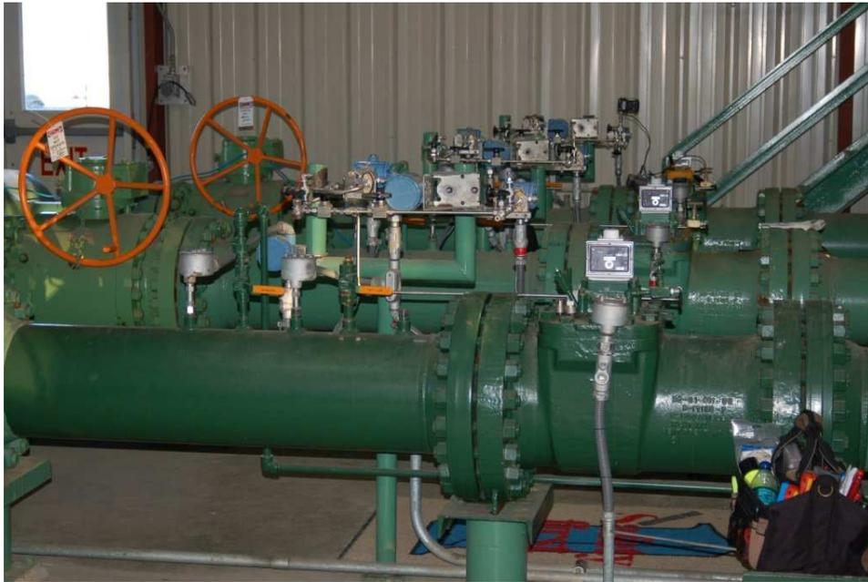
Note the pressure-sensing and temperature-sensing instrumentation installed in the pipe, reporting gas pressure and gas temperature to a flow-calculating computer (along with turbine pulse frequency) for the calculation of natural gas flow rate. Less-critical applications may use a “compensated” turbine flowmeter that mechanically performs the same pressure- and temperature-compensation functions on turbine speed to achieve true gas flow measurement, as shown in the following photograph:
