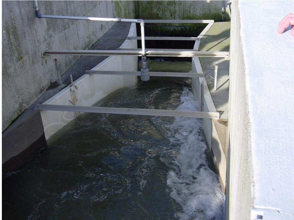
Once the liquid level is successfully measured, a computing device is used to translate that level measurement into a suitable flow measurement (and in some cases even integrate that flow measurement with respect to time to arrive at a value for total liquid volume passed through the element, in accordance with the calculus relationship  $V = \int Q dt + C$ ).
