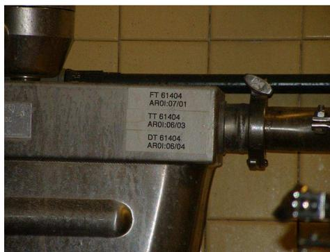
Even though a Coriolis flowmeter inherently measures *mass* flow rate, the continuous measurement of fluid density allows the meter to calculate *volumetric flow rate* if this is the preferred means of expressing fluid flow. The relationship between mass flow ( $W$ ), volumetric flow ( $Q$ ), and mass density ( $\rho$ ) is quite simple:
