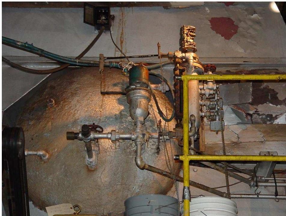
The switch mechanism is a mercury tilt bulb, tilted by a magnet’s attraction to a steel rod lifted into position by a float. The float directly senses liquid level, which positions the steel rod either
