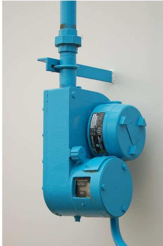
The spring reel's angular position may be measured by a multi-turn potentiometer or a rotary encoder (located inside the "head" unit), then converted to an electronic signal for transmission to a remote display, control, and/or recording system. Such systems are used extensively for measurement of water and fuel in storage tanks.
