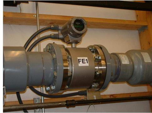
Other magnetic flowmeters have separate electronics and flowtube assemblies, connected together by shielded cable. In these installations, the electronics assembly is referred to as the flow transmitter (FT) and the flowtube as the flow element (FE):
