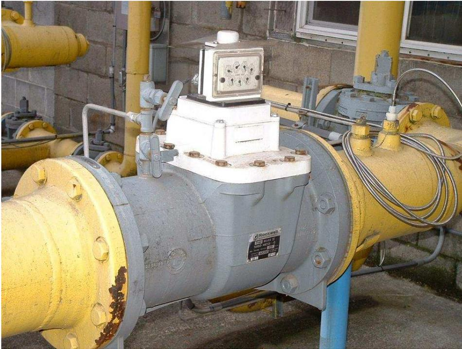
The particular flowmeter shown in the above photograph uses a filled-bulb temperature sensor (note the coiled, armored capillary tube connecting the flowmeter to the bulb) and shows total gas flow by a series of pointers, rather than gas flow *rate*.
