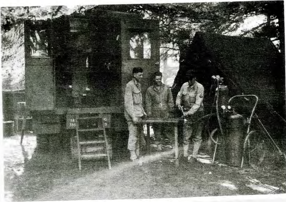
IN FRANCE THE REPAIR AND MAINTENANCE SECTION BUILT ITS FIRST LATRINE
