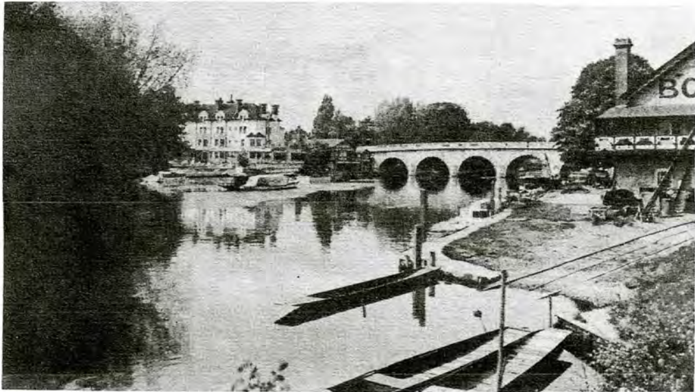
THE BRIDGE, MAIDENHEAD
